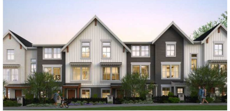
Street fronting townhouses (Image Credit: Gatehouse Developments)
