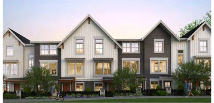
Street fronting townhouses (Image Credit: Gatehouse Developments)
